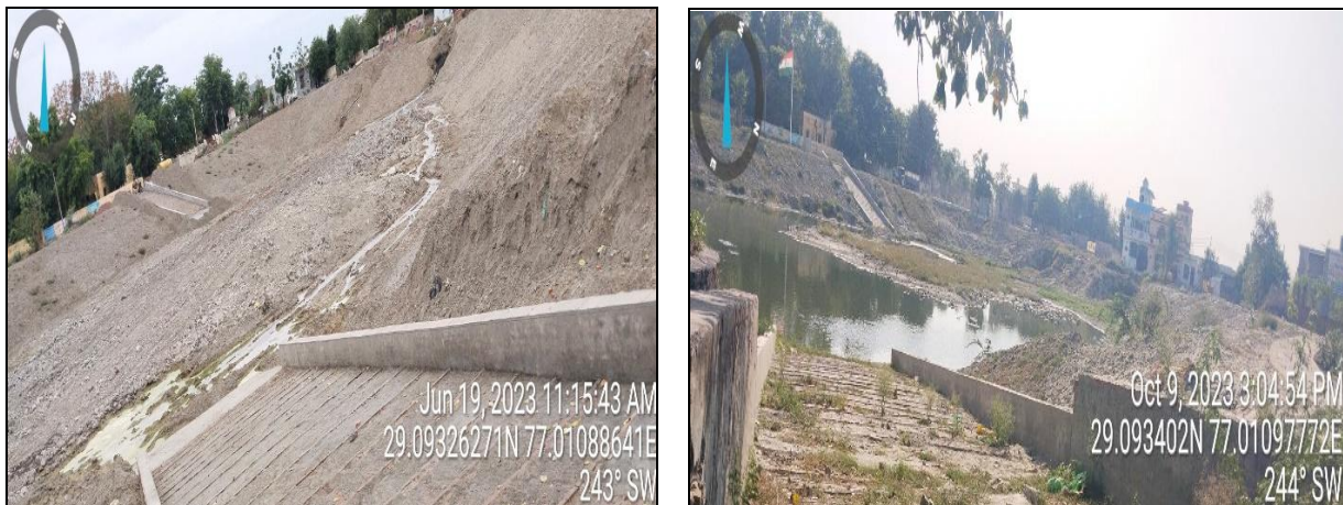
Photo 2: (a) Rajlu Pond during Rejuvenation work (b) After work Completion
