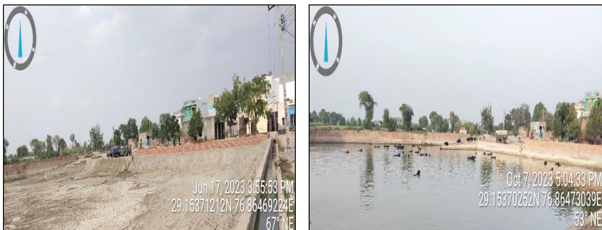
Photo 1: (a) Bajana Kalan Pond during Rejuvenation work (b) After work Completion
